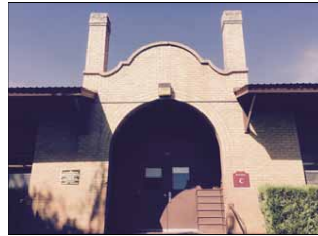
Close-up of the original Pearce Elementary School facade. The two chimneys are from a time when coal-burning stoves sat in each classroom.
