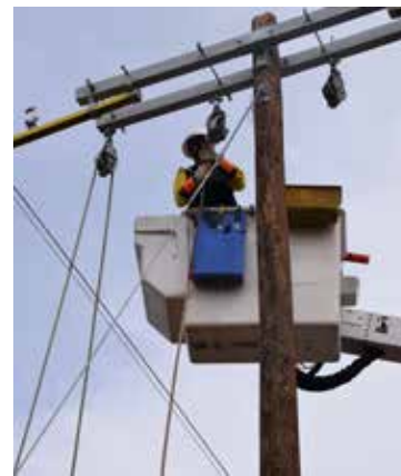
Dave Schmidt hanging stringing dollies.
