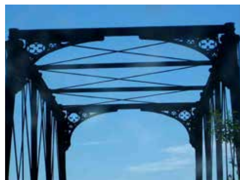
Overhead, we see none of the usual angle, channel, and H-beam structures now in use.
