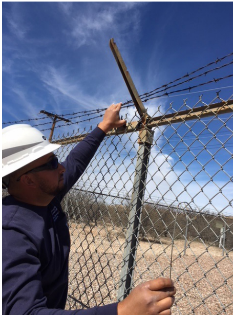
Reggie Morales, Apprentice Substation/SCADA Technician, tests the top guard of a substation fence.
