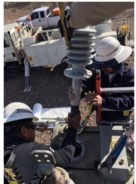
Ruben Nieto, Electrical Apparatus Foreman, and Felipe Mendoza, Journeyman Electrical Apparatus Technician, install a new bushing at the Tombstone Substation Transformer.
